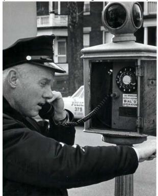
Photo showing the interior of Saint Louis Police Call Box with red light on top in 1962. The red light on top of the call box was activated when a call was pending. You could find anything stored in a call box when the door was opened. To call the desk you dialed 20, the captain dial 22, the detective bureau dial 24, the report room dial 25 or 26, the juvenile office idal 24 or 28, and to dail another district 9 + 5 + one of the numbers above.
